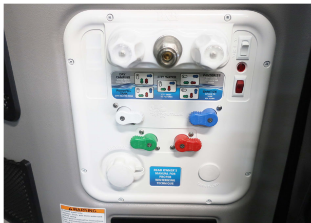
Water Center Panel in “Winterize” configuration (Panel located behind passenger rear door) -Typical view
